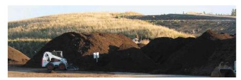
Figure 23. Composted greenwaste piles (brown, foreground) will be used as a soil amendment. After the landfill has been covered with soil (right, background) it is seeded with grass (left, background)
