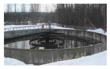
Figure 19. More solids settle out in large tanks (clarifiers).
