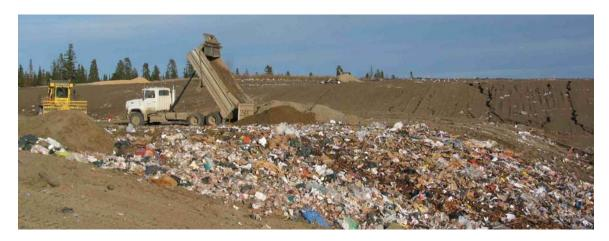
Figure 22. Compacted garbage is ready for a cover of soil. The dumped soil will be spread across the garbage to create a refuse cell. The soil-covered slope in the background is underlain by many refuse cells.
