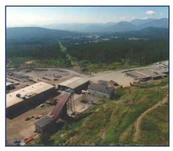
metal sulphide was shipped by train to the smelter in Trail where zinc, lead, and silver metal was produced. Fine waste rock or tailings were stored in large storage ponds behind low dams. Waste rock was dumped in piles near the mine entrances.
