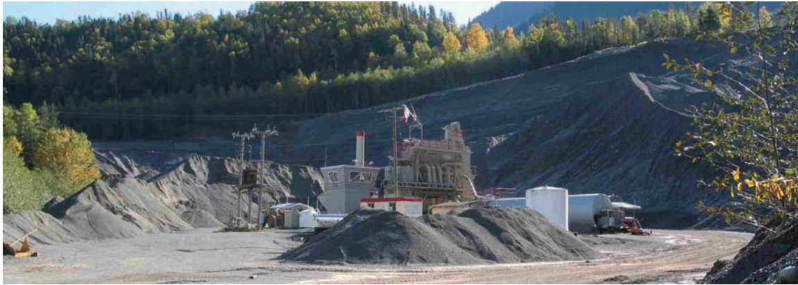
Figure 28. Asphalt plant on along Highway 16 east of Thornhill. Sand and gravel are quarried from Ice Age deposits, sorted, and combined with liquid asphalt at the plant.
